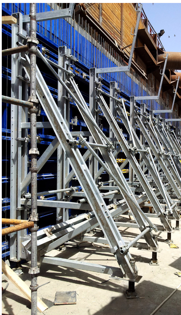
Modular supporting unit formed by combining attachable frames of 1.50m
